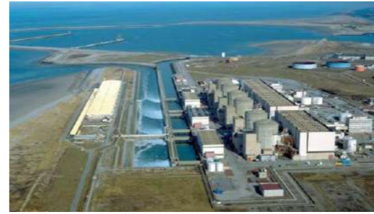
Nuclear Power Plant (Gravelines + Normandy)
